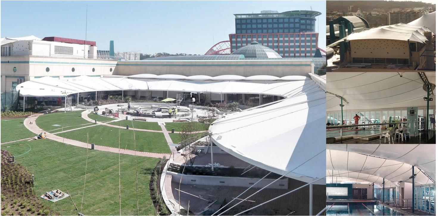
The roof of the Colombo Shopping Centre was built over an already existing swimming pool, with a covered surface area of 3,100m<sup>2</sup>. The main condition required in the design was simple dismantling of the structure.
